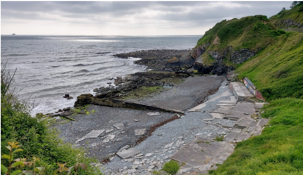
Figure 1 – CCA5-A: The sub-cell is made of a series of natural rock faces and coves/beaches. The image here shows Naylor's Cove, the most northerly cove in the sub-cell. Remains of old stairs and baths are present and provide coastal protection, with a rocky foreshore and steep grassed slopes above.
