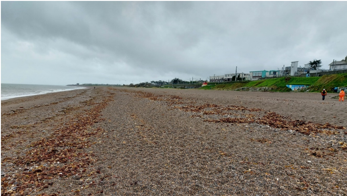
Figure 1 – CCA6.1-A: The sub-cell is a 1km long shingle beach, located at the front of Greystones station. The beach is 100m wide beach and has varying height levels depending on storm conditions. Vegetated embankments and concrete retaining walls are located at the back of the beach.
