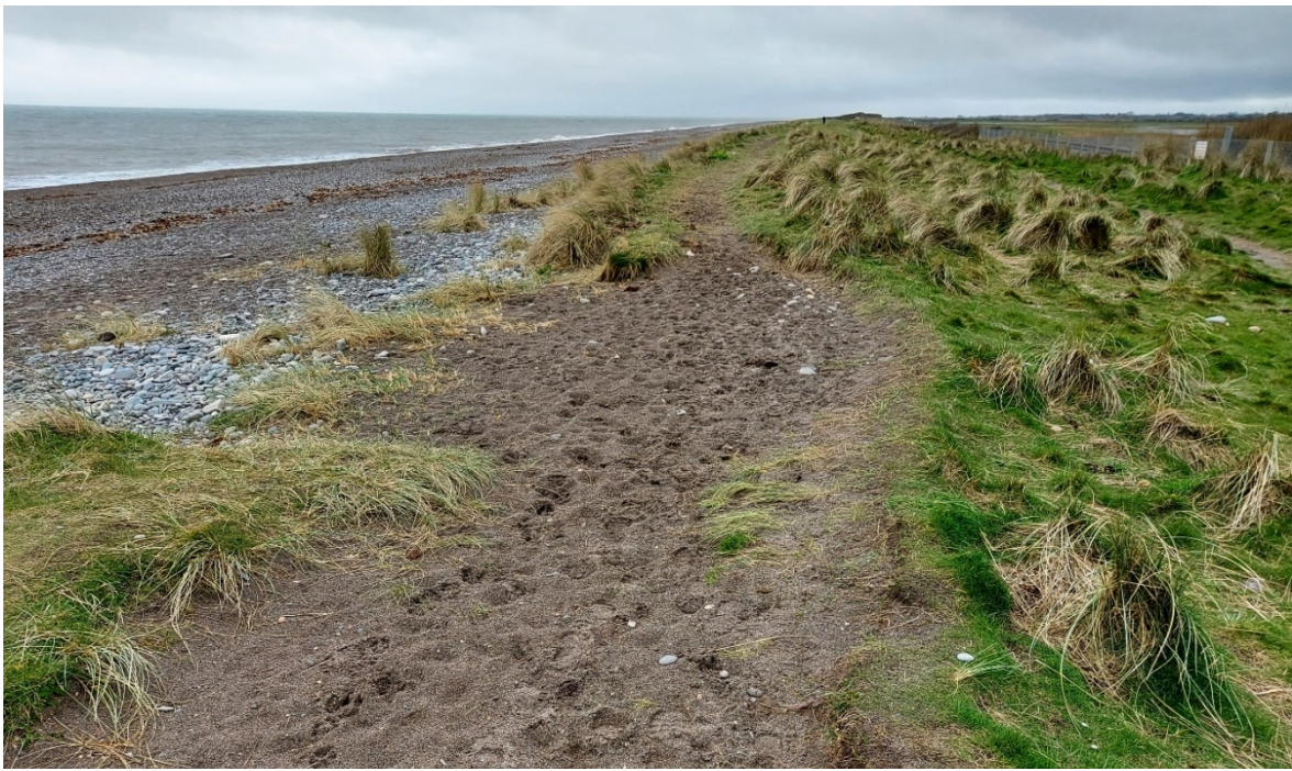
Figure 5 – CCA6.1-D: The sub-cell here has a 60m wide sand-shingle mix beach, with low vegetation at the back of the beach. Evidence of local erosion due to wave action is visible, highlighting the increasing impact of storms on the beach.
