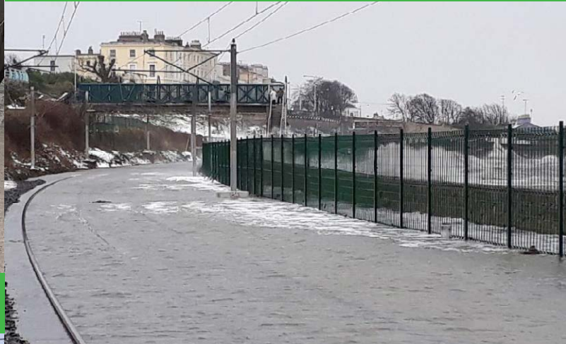
DART line coastal flooding, March 2018
