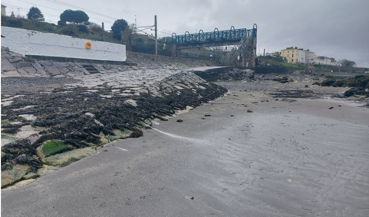
Figure 11 - CCA1-E: Through the sub-cell, the defence is made of a sloping masonry revetment with upstand wall. In this area, a sand beach and rocky foreshore is located at the front of the engineered asset. A walkway runs along the sub-cell.
