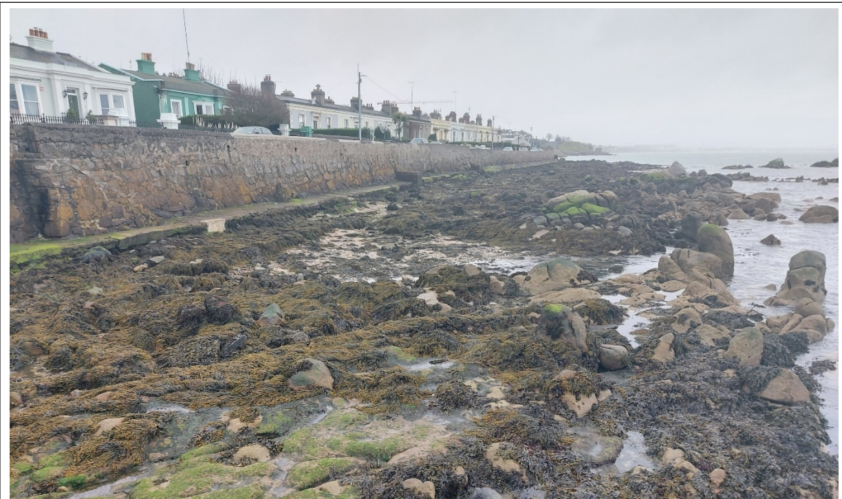
Figure 9 - CCA1-D: At the far end of the sub-cell, Brighton Vale is a series of 15 properties located between the railway and the foreshore. There is a continual wall alongside the railway protecting the line.
