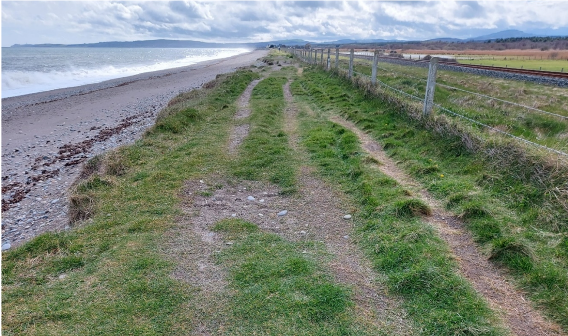
Figure 1 – CCA6.2-A: The first half of the sub-cell is a 1.5km long beach, with an approximate width of 40m. The beach is a sand and shingle mix, backed by low vegetated strip. The railway is approximately 15m behind the boundary fence, but evidence of erosion is visible at the edge of the vegetation.
