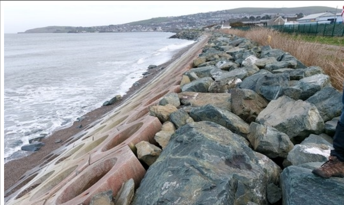
Figure 5 – CCA6.2-E: The last 200m of the cell consist of a recently built engineered coastal defence, with sloped interlocked concrete blocks, and rock revetment at the crest. Beaches levels have been eroding rapidly in this area, but the presence of land at the back of the beach provides additional buffer.
