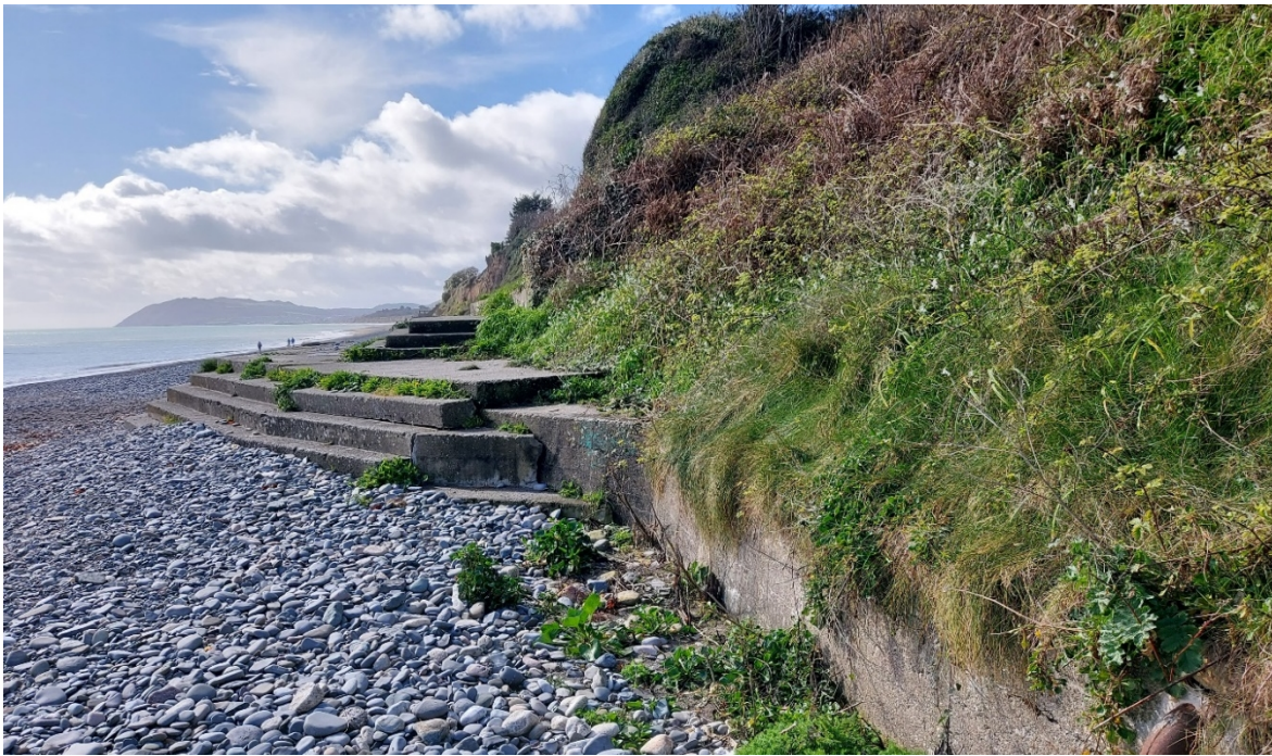
Figure 7 – CCA2/3-C: The rest of the sub-cell is made of the same coarse material beach, with a half meter high upstand wall and vegetated cliffs. Killiney station is located shortly after these concrete stairs and is located at the top of a steep vegetated cliff.
