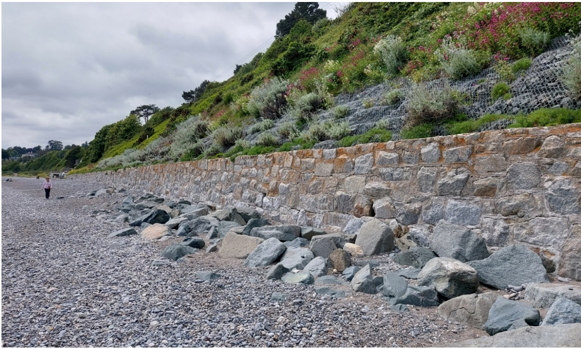
Figure 5 – CCA2/3-B: The rest of the sub-cell is protected by a 3m high masonry wall, with gabion baskets at the top and small boulders at the bottom. The picture here is taken just after Whiterock Beach outcrop and shows the beach widening in the western direction (left hand-side on the image).
