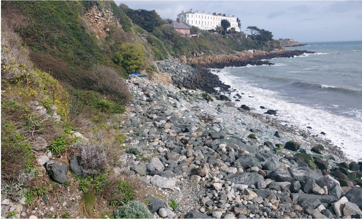
Figure 1 – CCA2/3-A: The eastern end of the sub-cell is made of a 200m long beach, with steep vegetated cliffs and placed rock protecting the base of the cliff. At the west of the beach, the Vico Baths are located at the bottom of a rock outcrop and are made of a series of concrete steps and rails.
