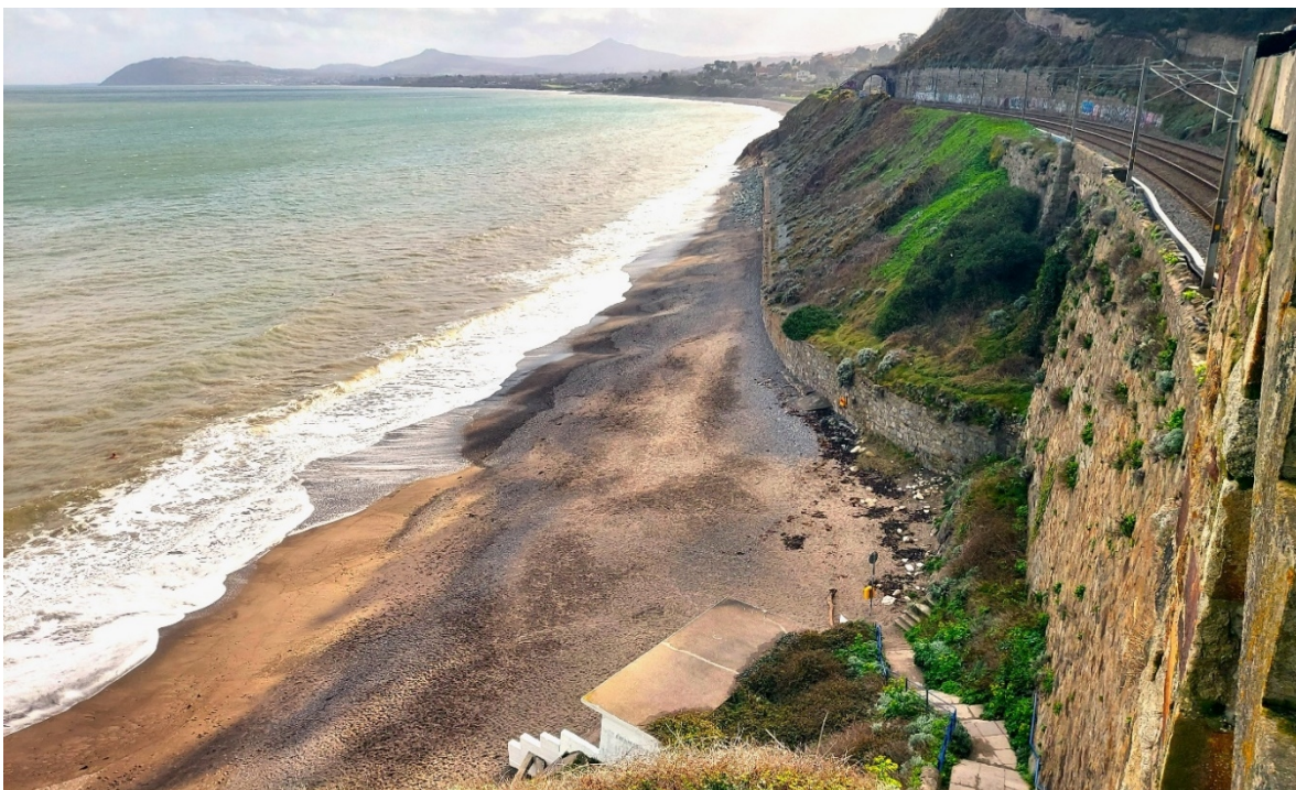
Figure 4 – CCA2/3-B: This sub-cell is the northern part of Whiterock/Killiney Beach. A 25m high retaining wall can be seen on the right-hand side of the image. Whiterock rock outcrop is also visible where the beach narrows, with some boulders on the beach. A smaller wall is also located between Whiterock outcrop and the 25m high retaining wall, with gabion baskets at the crest.
